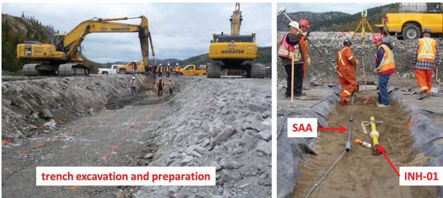
Figure 3. Installation of INH-01 and SAA.
